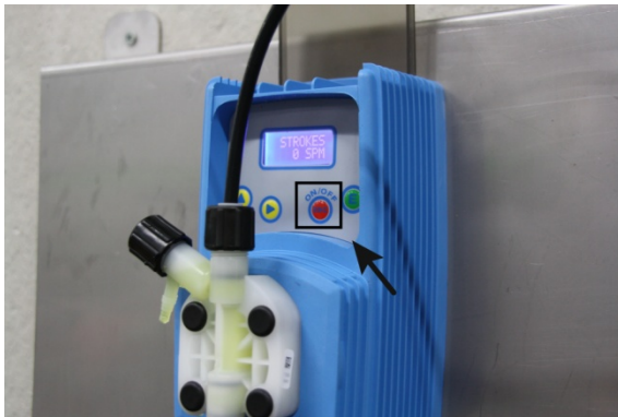
Figure 8: Switching the pump on
