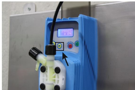
Figure 11: Filling the pressure hose
