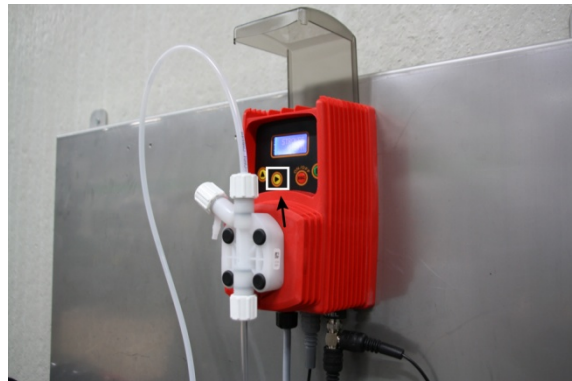
Figure 15: Filling the pressure hose
