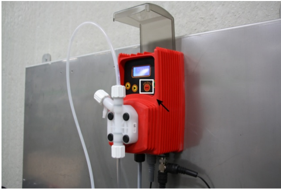
Figure 12: Switching the pump on
